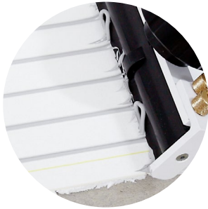
Direct bonding of FRP
